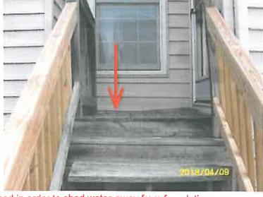
Marginal Grading: Needs to be properly raised in order to shed water away from foundation
