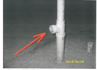
Unsatisfactory Unsatisfactory Cleanout Caps - loose and needs sealing at water main area CSST Type Gas Lines Needs to
